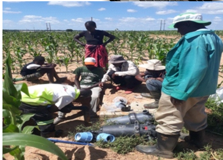
Drippers being installed in Tier 1.3 maize field by Water User Group members
